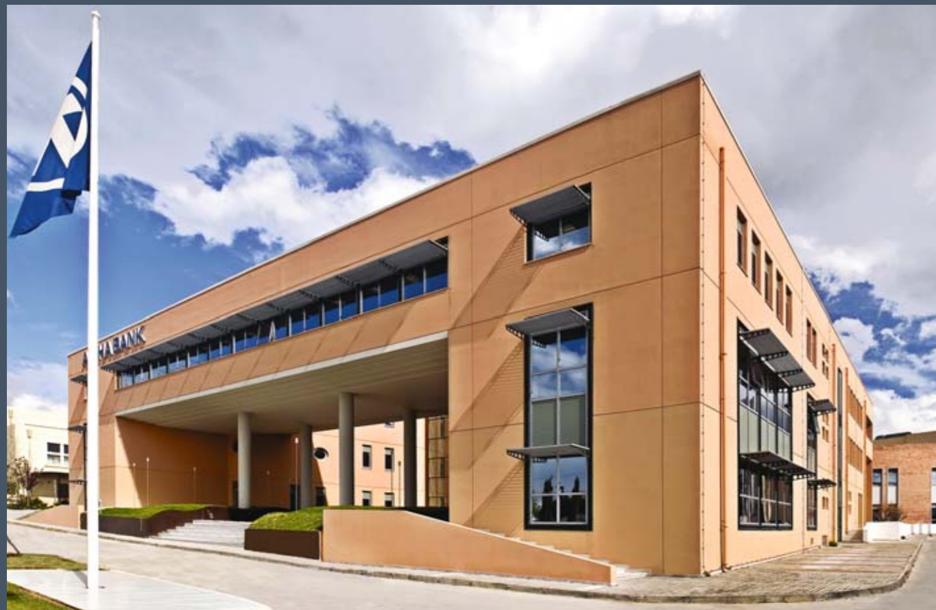
The facade of the first building (Building A), currently housing the Training Centre of the Bank.
